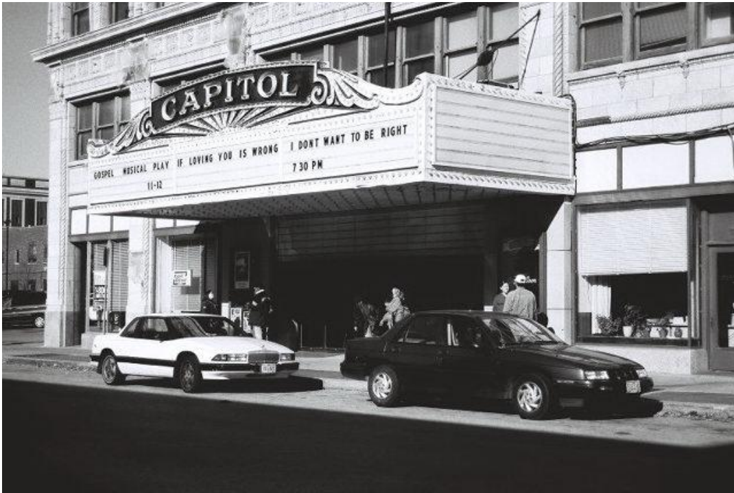
Detail view of the Capitol Theatre marquee located on the building's south elevation. An image of the historic canopy can be found in the Richardson-Sloane Special Collections of the Davenport Public Library (Image #VM89-000195). Regretfully, it is not included here.
