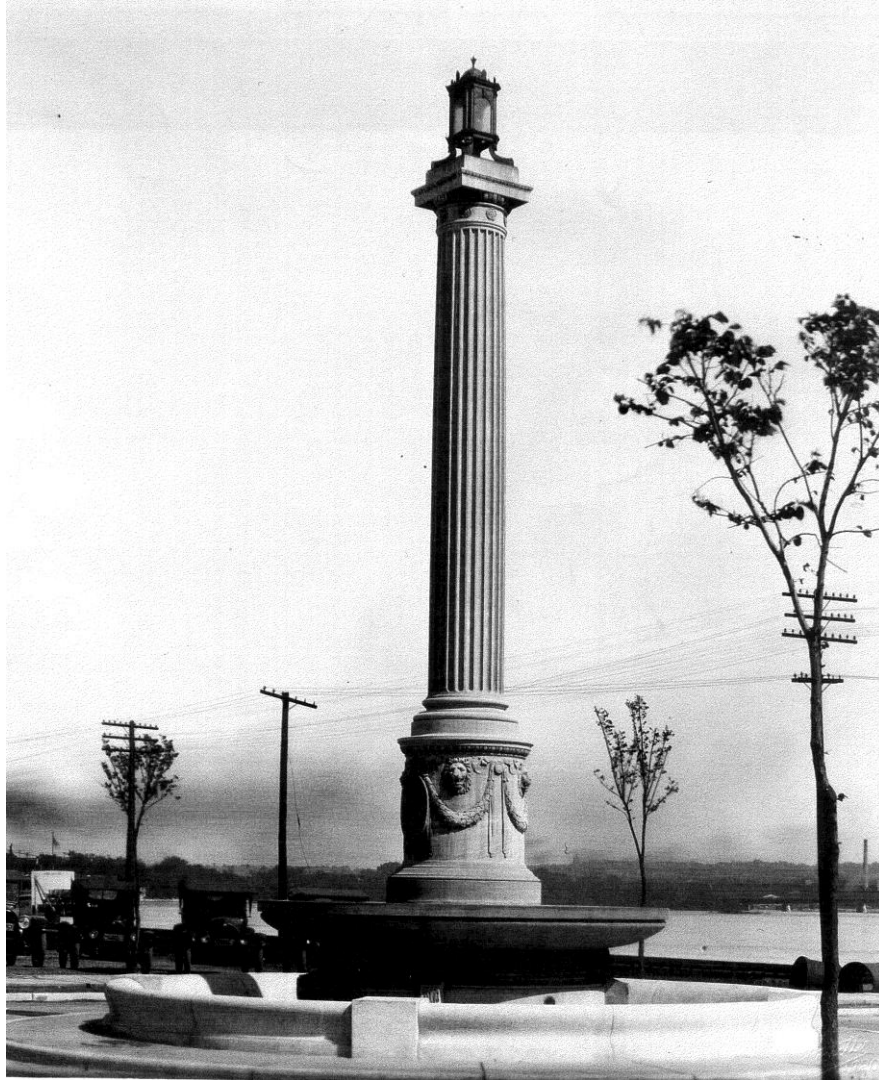
This c.1918 image documents the memorial shortly after it was erected in 1916.
