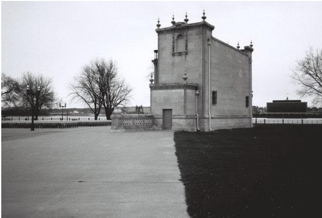
View of the rear elevation, looking south from near Beiderbecke Drive.
