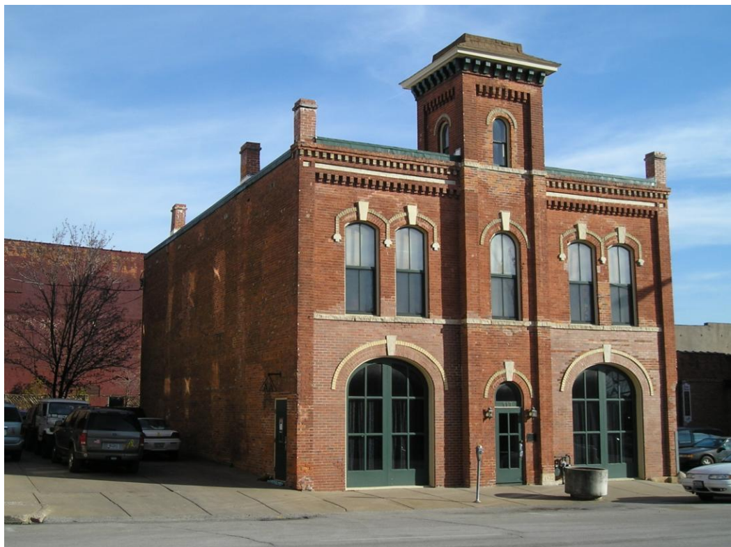
View of the primary (west) and north elevations, looking southeast across Pershing Street.
