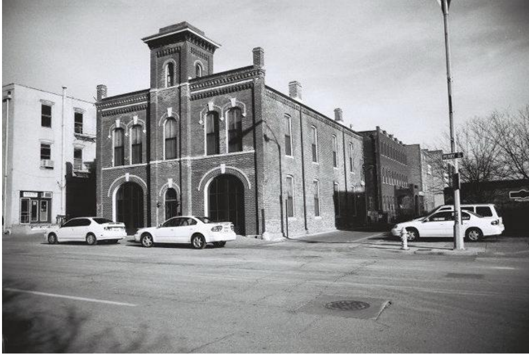
View of the primary (west) and south elevations, looking northeast across Perry Street.
