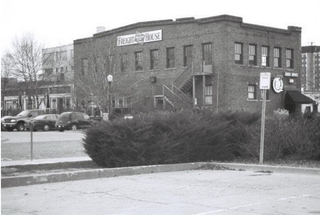
View of the east section of the structure, looking northwest across South Ripley Street. The one-story portion of the freight house building is seen here on the left.
