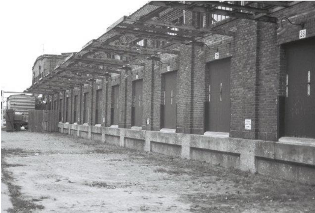
View of the loading docks on the West River Drive side.
